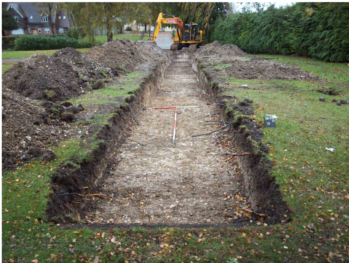
Plate 29: Trench 6 looking west-south-west
