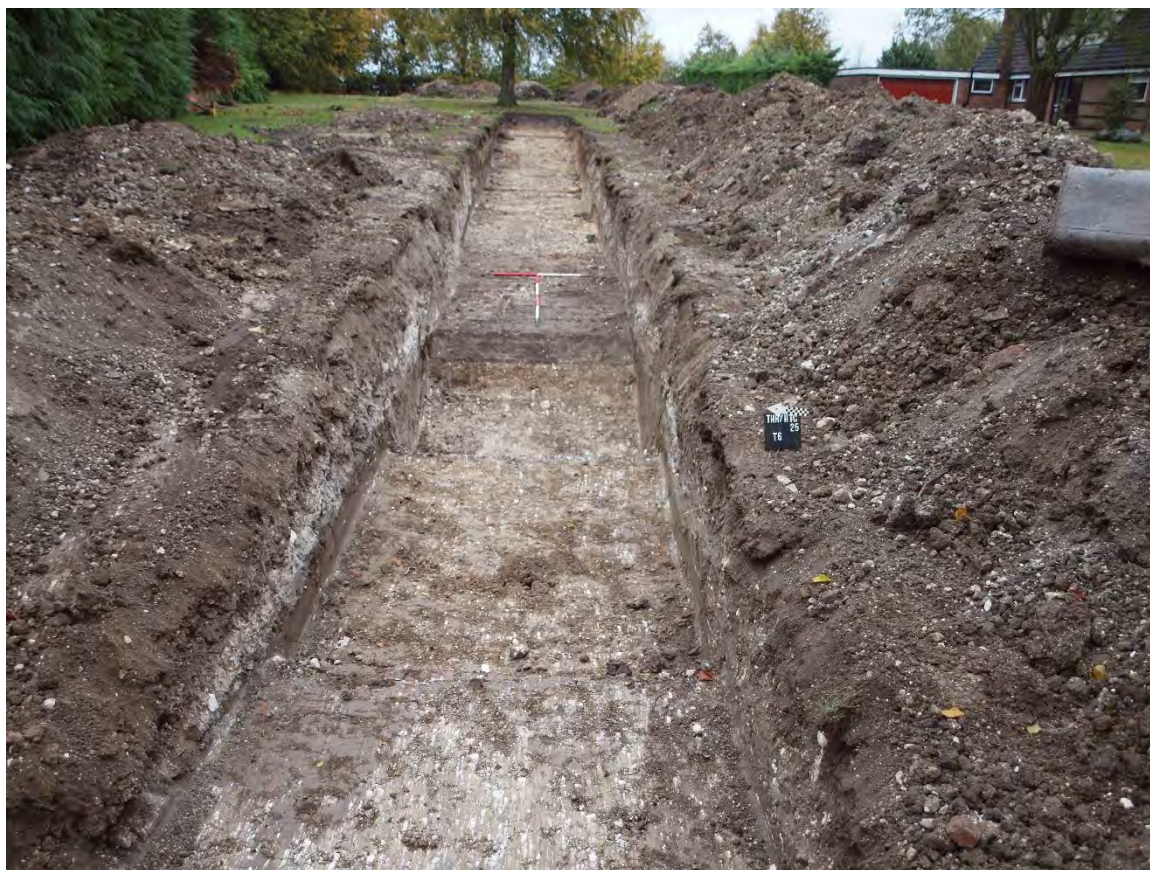
Plate 30: Trench 6 looking east-north-east
