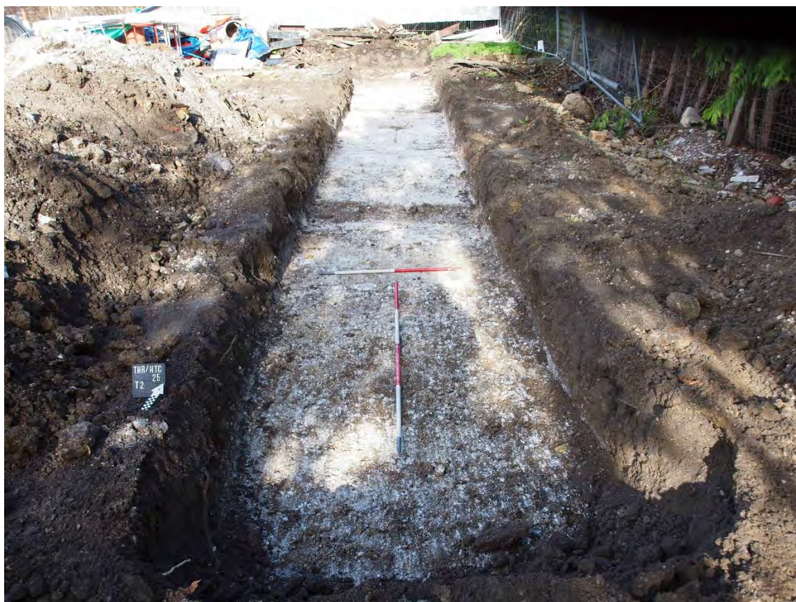
Plate 10: Trench 2 looking south-south-east
