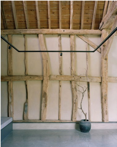
Exposing & Insulating Existing Structures - Hunts Green Barn by McLaren.Excell
