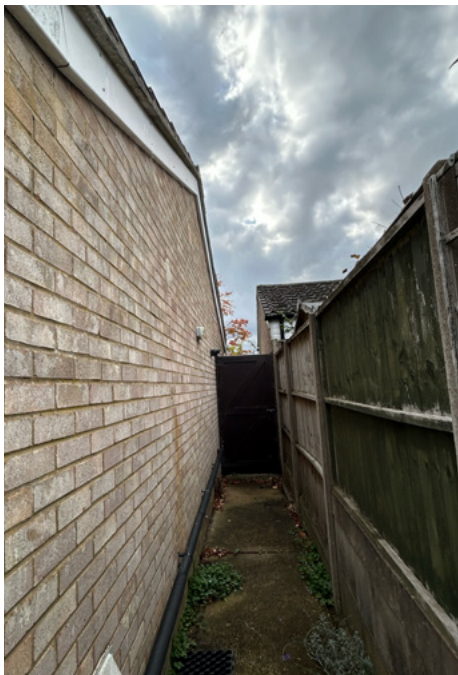
Side Facade (North-West) View from rear garden
