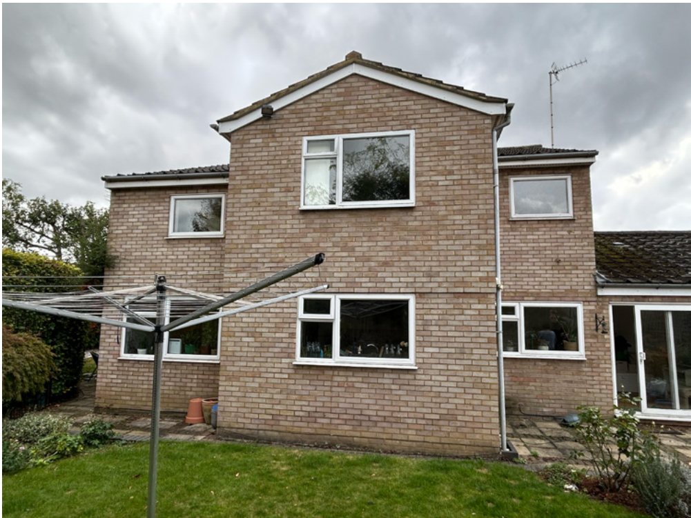
Rear Facade (North-East)
