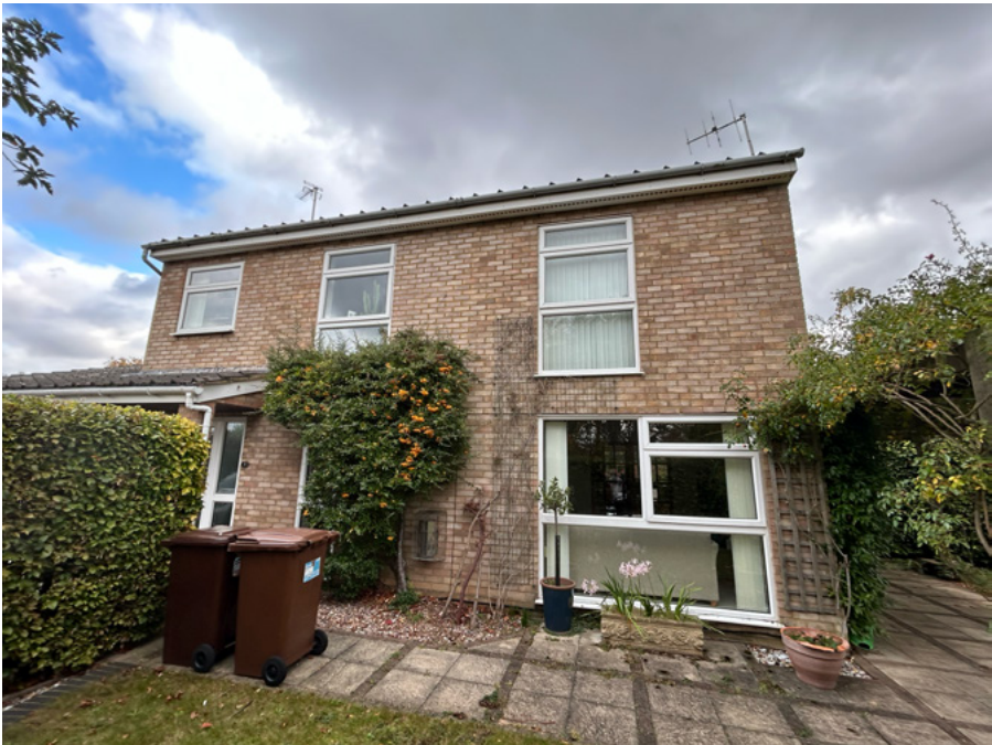
Front Facade (South-West) View from garden
