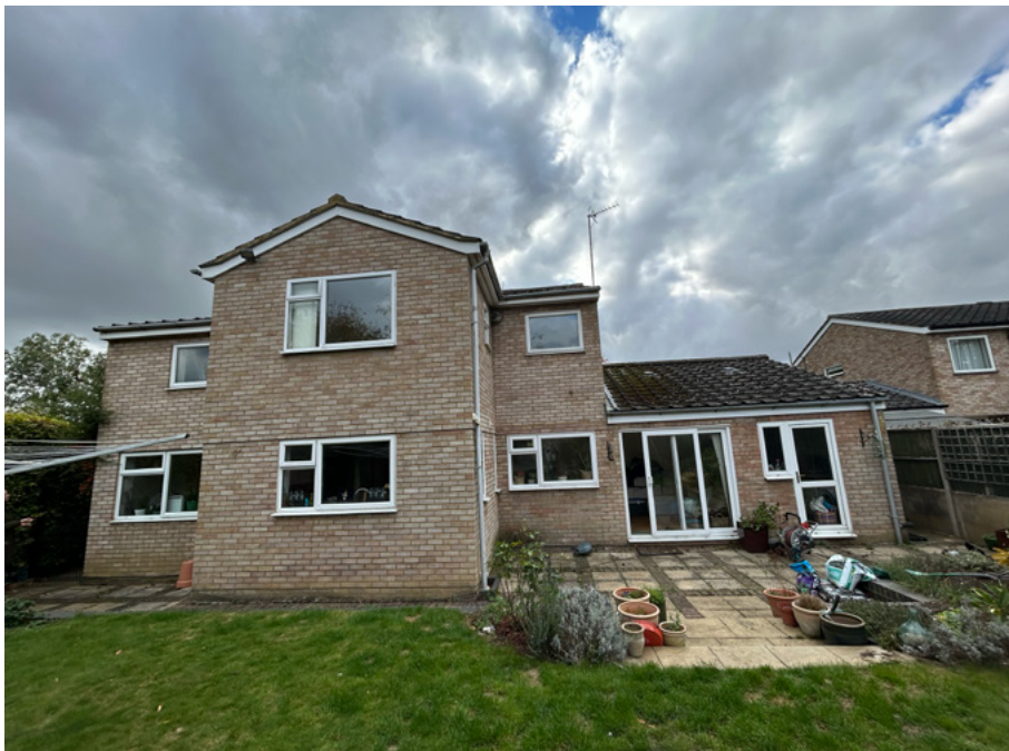
Rear Facade (North-East) View from rear garden
