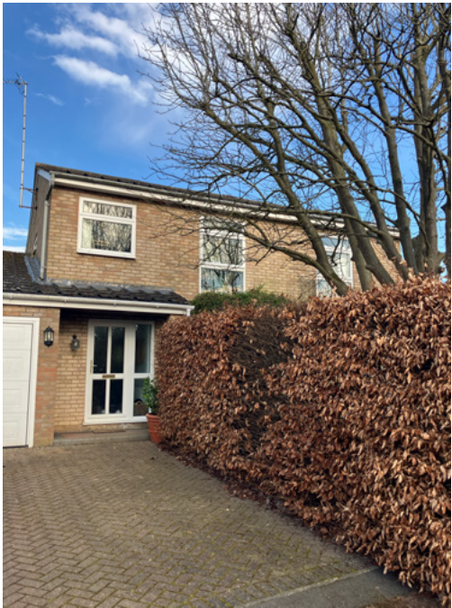
Front Facade (South-West) Approach view from driveway
