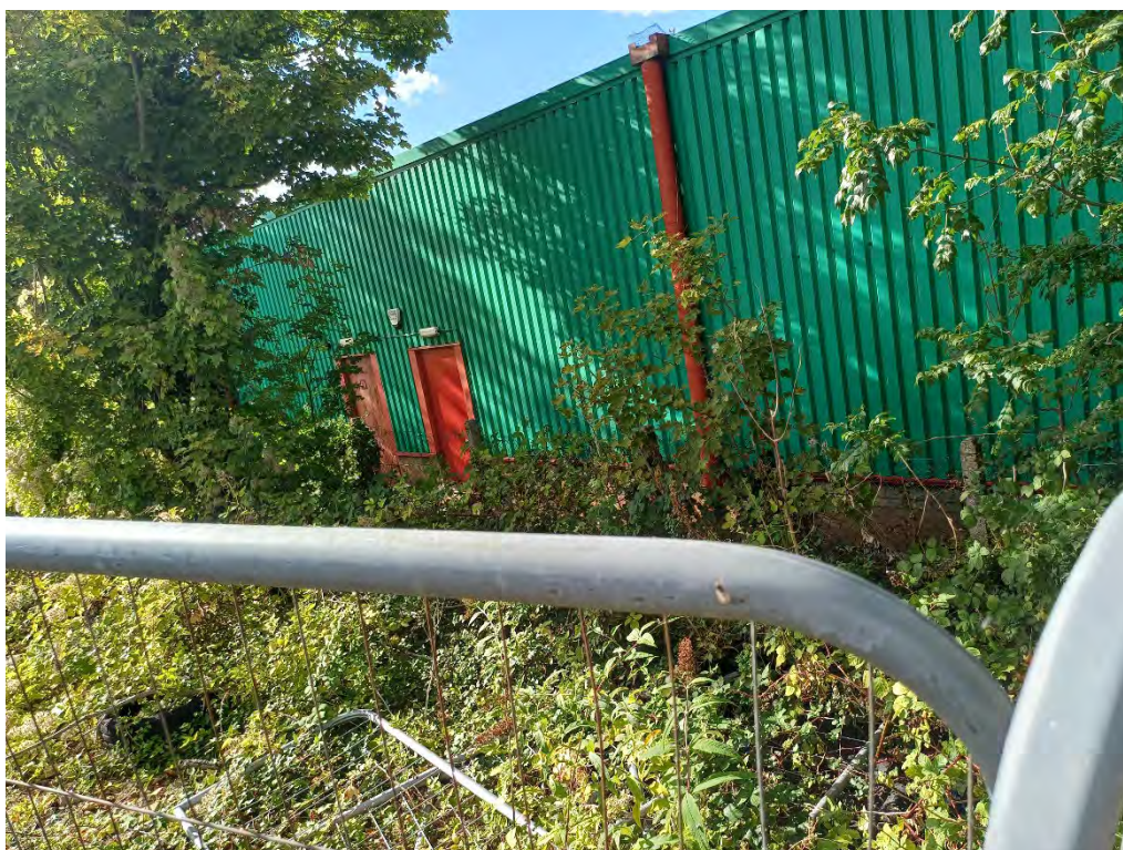
Photograph 08: View of Site, October 2025. Photograph Provided by Wedgewood Groundworks
