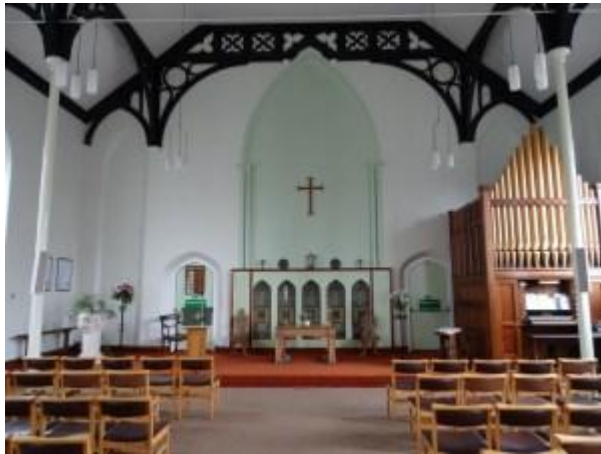
Nave showing alter roof truss and organ
