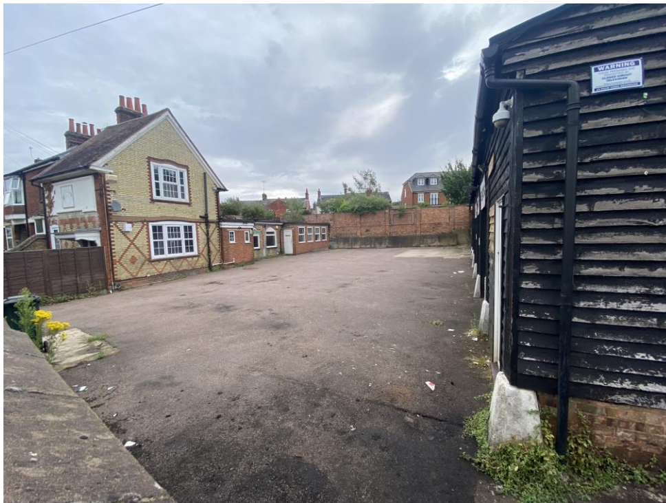
Photo 1: Looking northward towards 81a.
