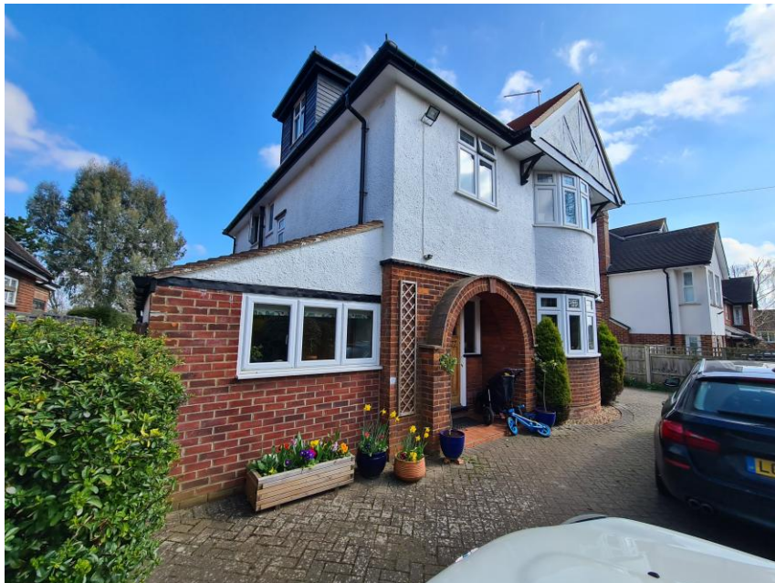
Fig 1: Existing front elevation of property
