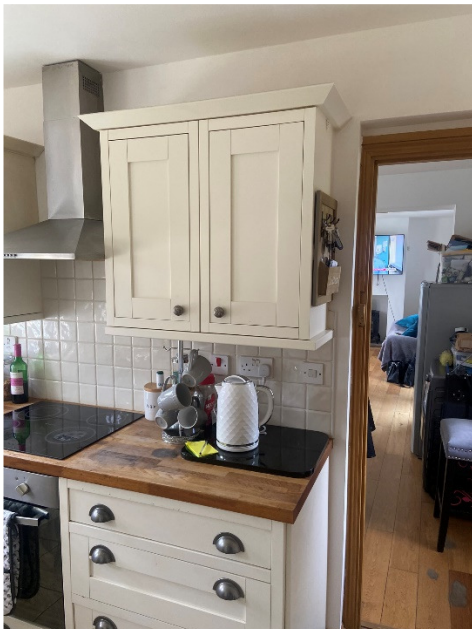
Kitchen wall to be removed
