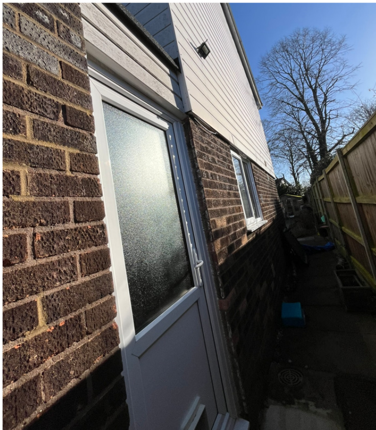
Existing right hand side access
