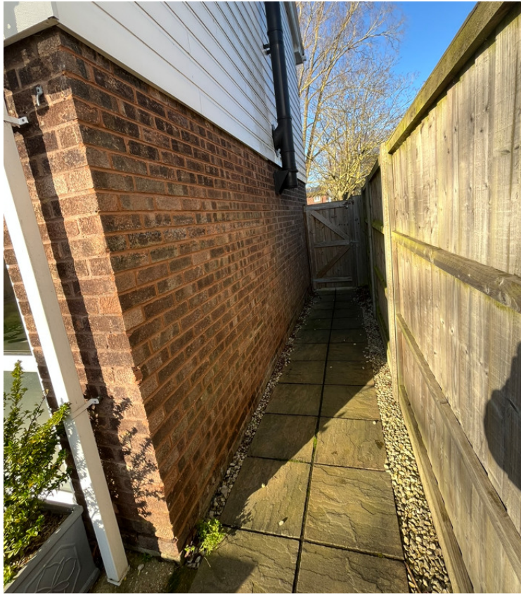
Existing right hand side access
