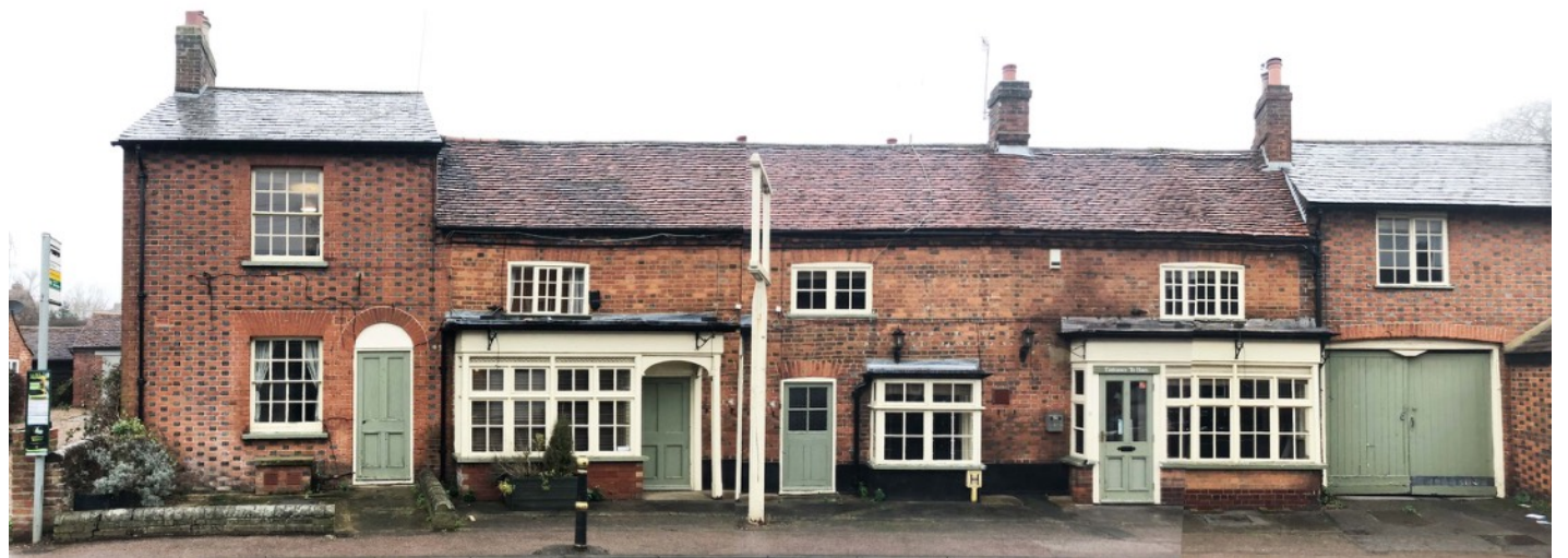
The White Horse, Kimpton Condition Report December 2024
