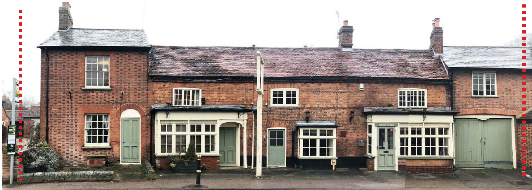
Existing Front (South) Elevation along Kimpton High Street
