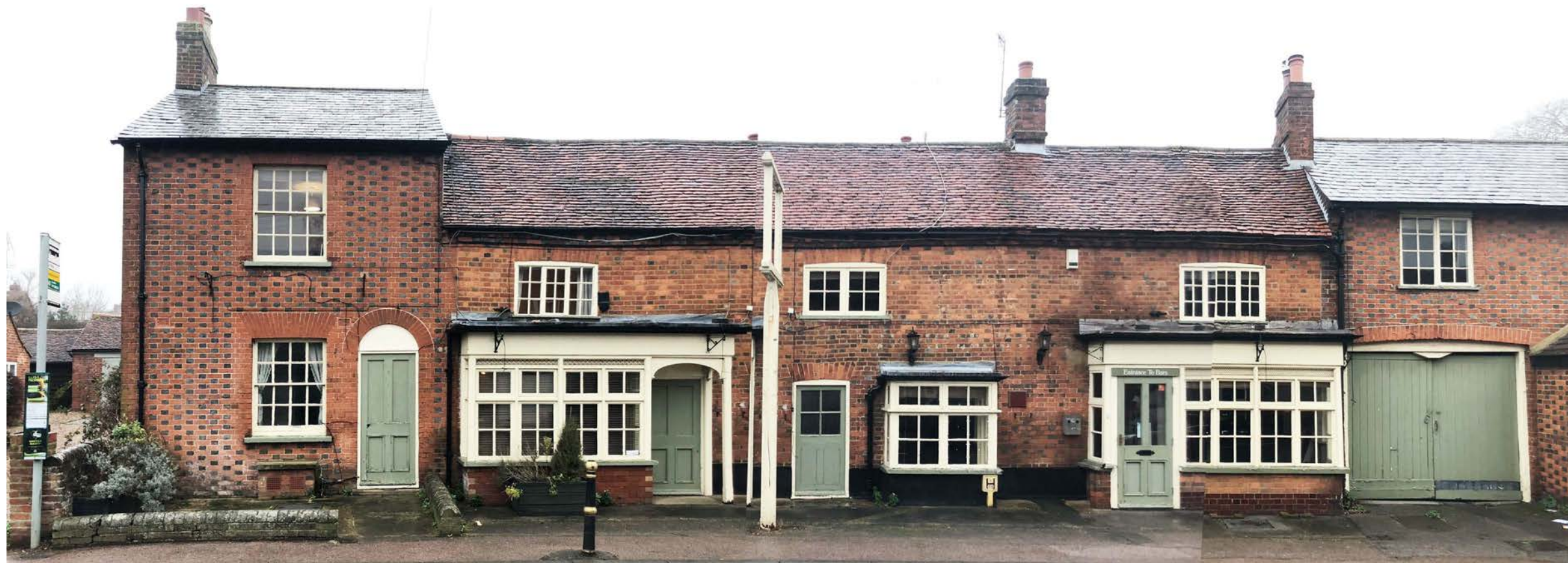
Existing front (south) elevation along high street
