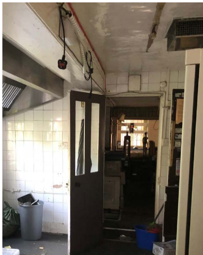
View of the rear kitchen (structural opening to existing rear wall visible)
