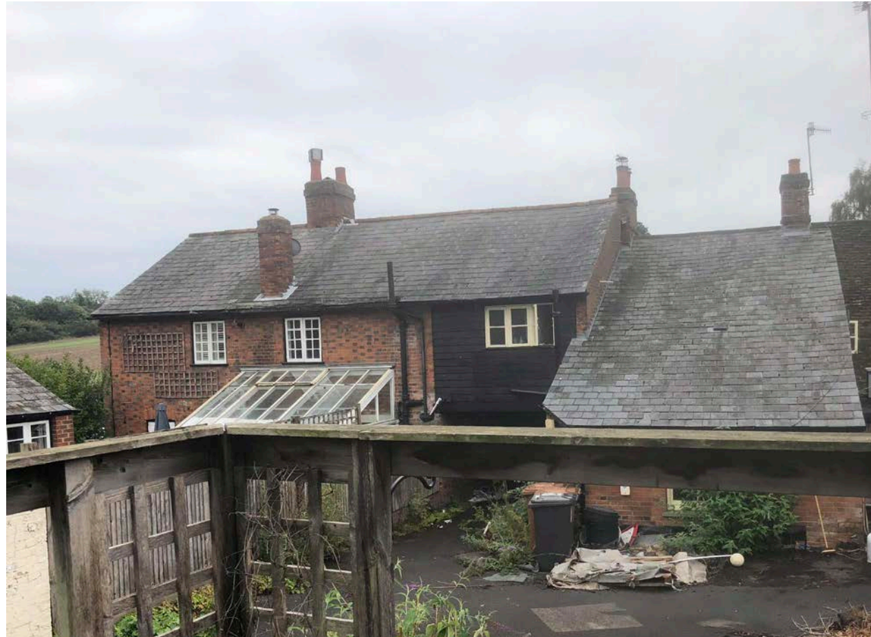
Existing Rear (North) Elevation -looking toward the south east
