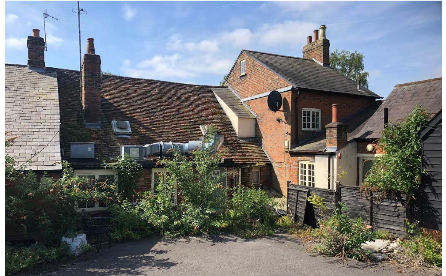
Existing Rear (North) Elevation -looking toward the south west
