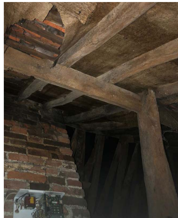
Existing timber trusses and posts within the main roof
