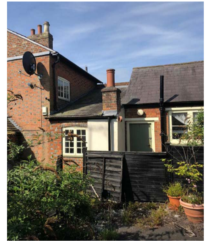
View of the rear return along the west boundary
