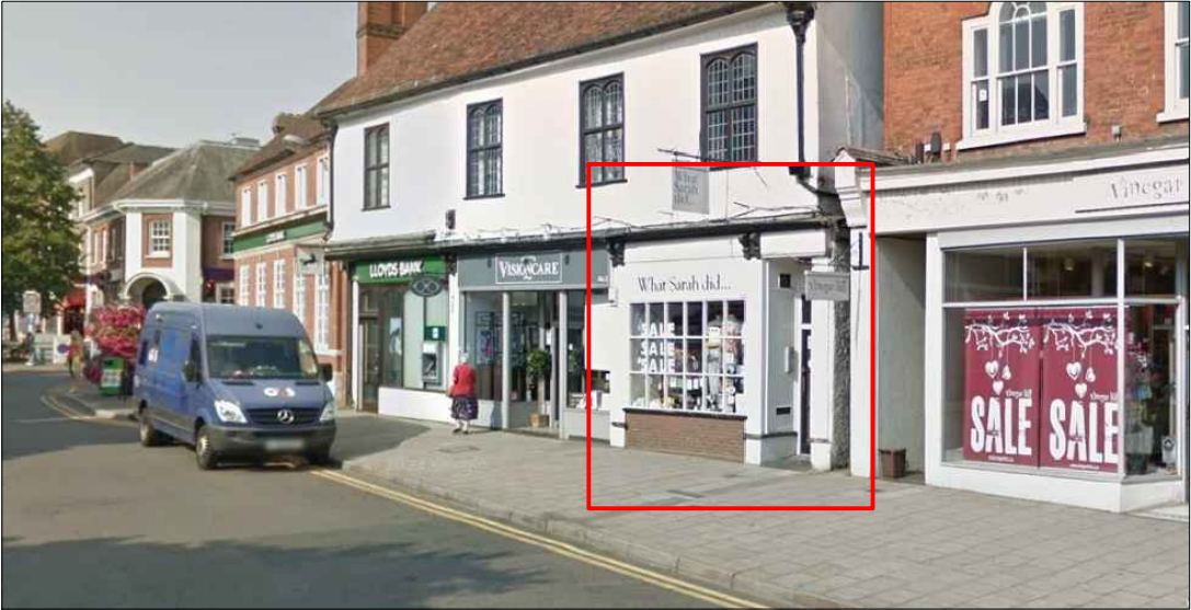
PRE-EXISTING FRONT ELEVATION - JULY 2018
