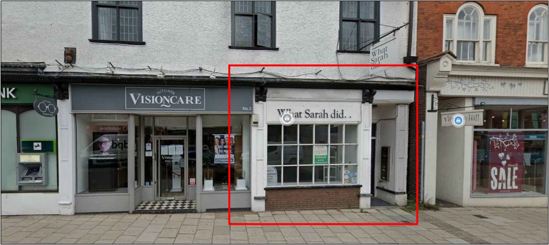
PRE-EXISTING FRONT ELEVATION - AUG.2020
