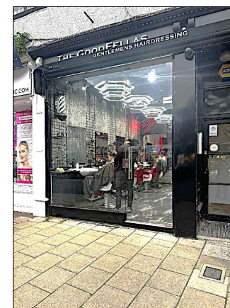
EXISTING FRONT ELEVATION - NOV.2024 Existing images of host building at 4 Bancroft consisting of an aluminium framed shopfront with aluminium paneled pilasters and stallriser with powder coated finish in jet black RAL 9005
