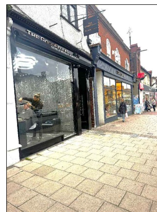
EXISTING FRONT ELEVATION - NOV.2024 Existing images of host building at 4 Bancroft consisting of an aluminium framed shopfront with aluminium paneled pilasters and stallriser with powder coated finish in jet black RAL 9005
