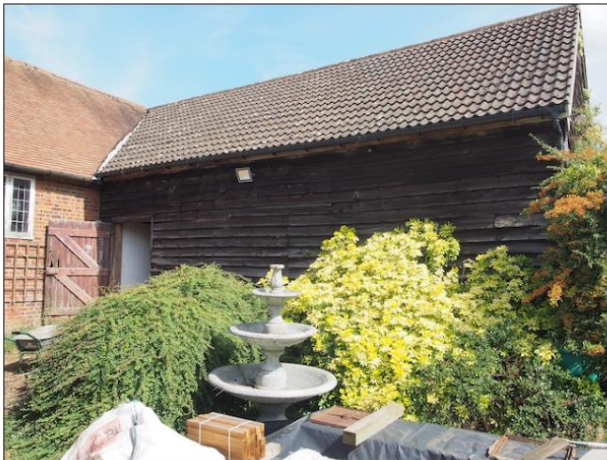
Photo 11: Internal (rear) elevation of the cart-shed
