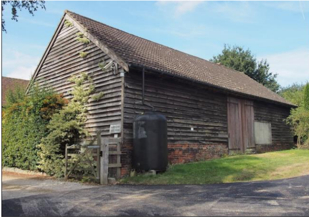
Photo 9: Front elevation of the former cart-shed fronting the road
