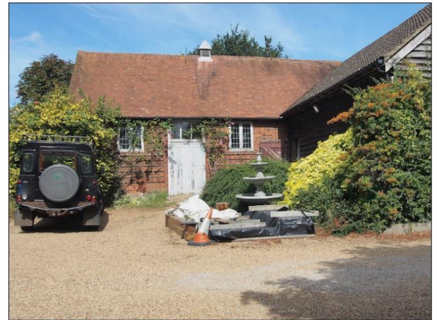
Photo 12: Front and gable elevation of the former stables
