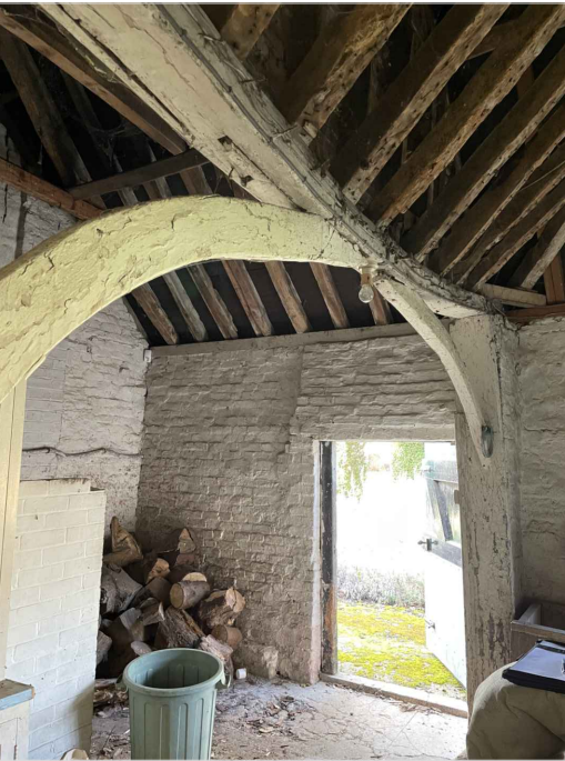
Photo of existing timber brace in store
