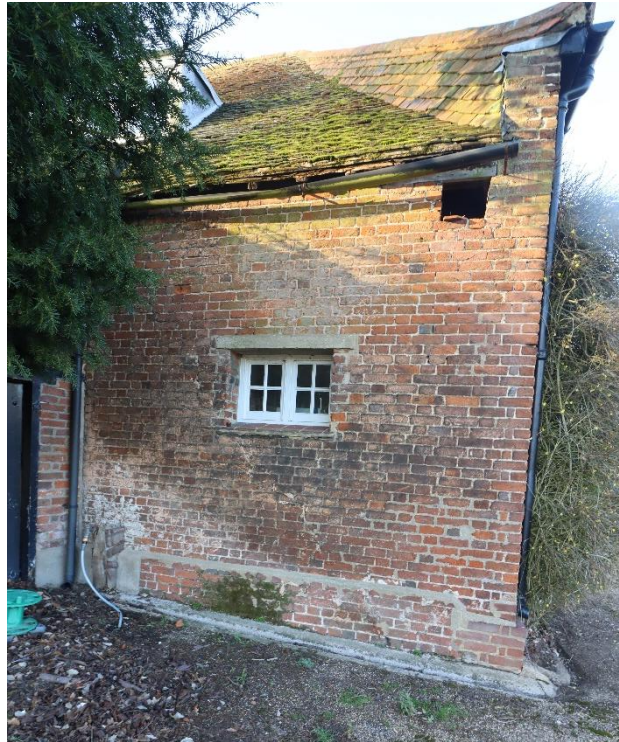
South-east corner of former Coach House
