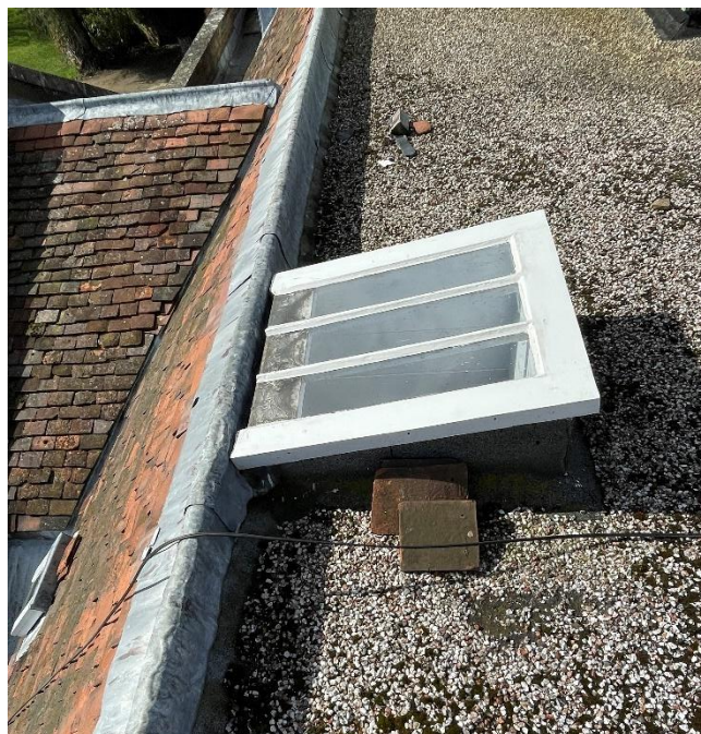
Rooflight R3 located against upstand kerb
