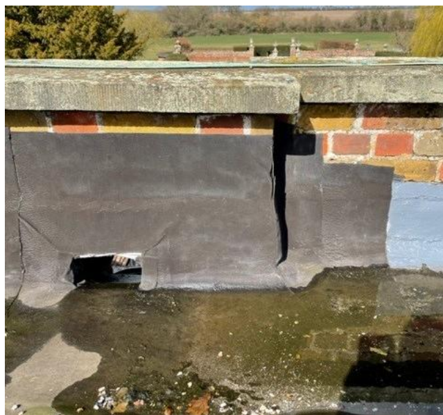
Villa flat roof outlet to north parapet wall
