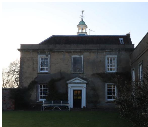
Lead chute to right of east tiled roof
