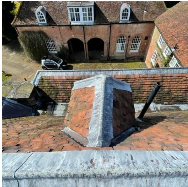
Dormer window to second floor west side bathroom
