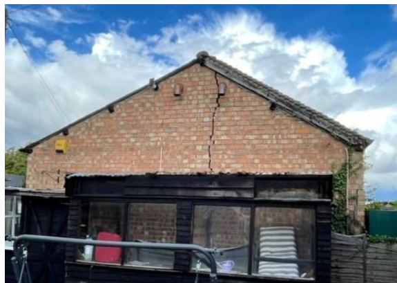
South wall of outbuilding
