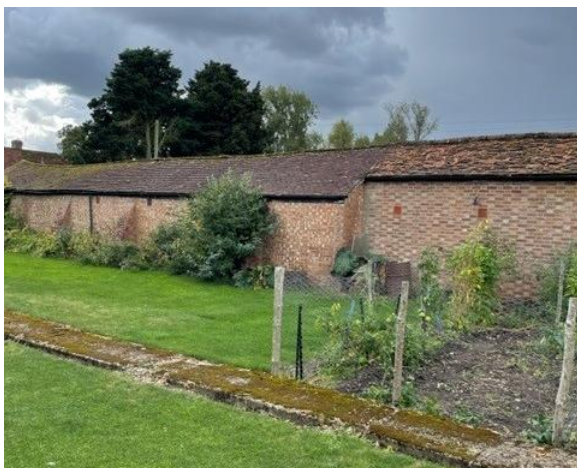
East elevation of outbuilding
