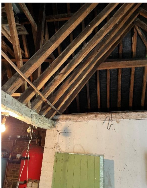
Existing Boiler Room. MC20th partition and door forming workshop to be removed. Historic rafters to remain.
