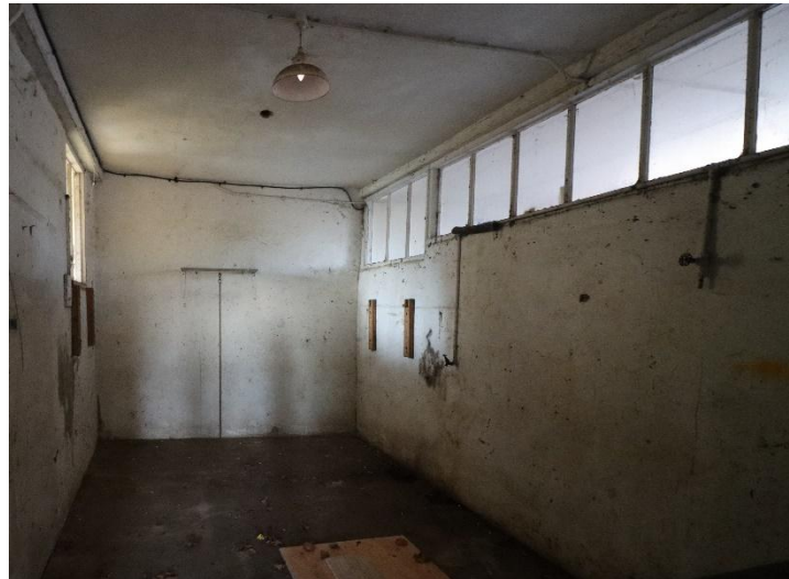
C20 th partition to be removed (rhs)
