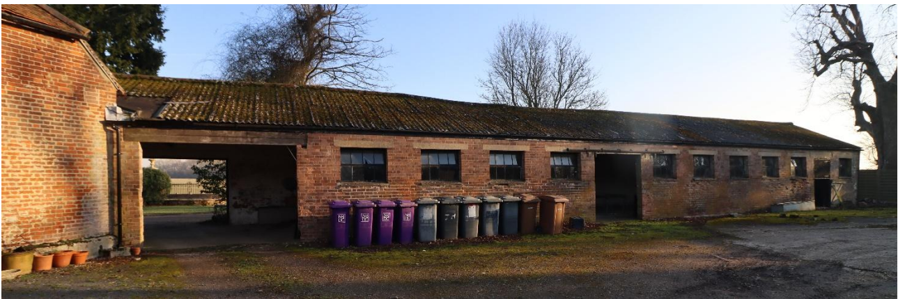
MC20 th garages (north-west elevation)
