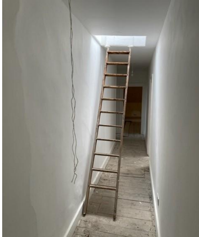
Existing MC20 th fixed ladder to be removed. Construction materials of ceiling to be confirmed.
