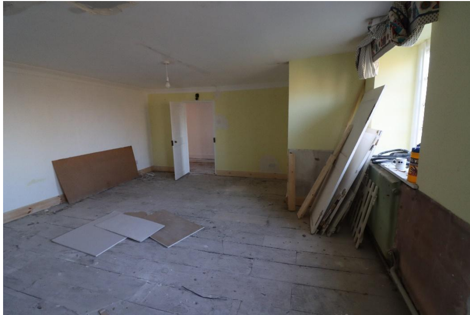
MC20th WC partitions to be removed (rhs)
