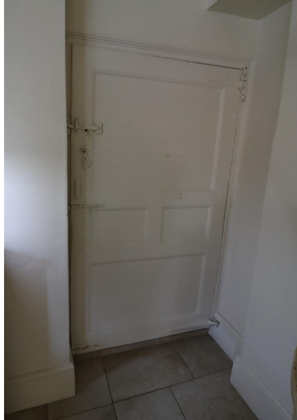
Georgian door (Historic Recording P20) to be relocated to form lobby to Master Bedroom suite
