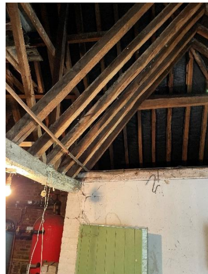
Brick pier and workshop partitions to be removed
