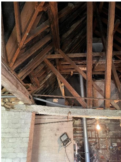
Brick pier and workshop partitions to be removed
