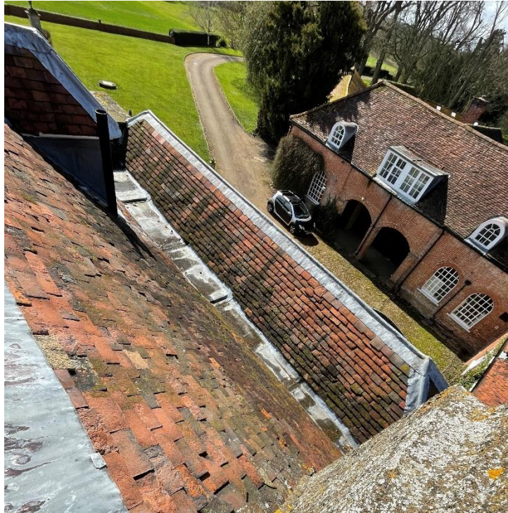
View to lead stepped valley gutter and tiled dormer window to 2 nd floor bathroom (west side)
