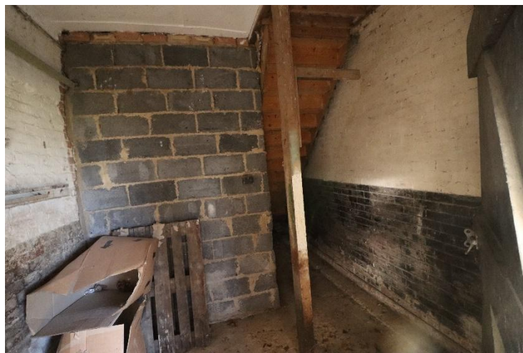
Blockwork partition to be removed and approx location for proposed new door opening (rhs)
