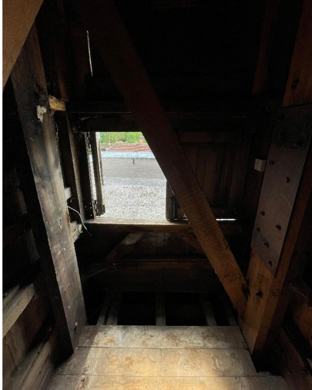
Inside of clocktower view out through doors
