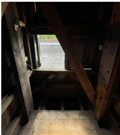
Bracing within the body of the clocktower
