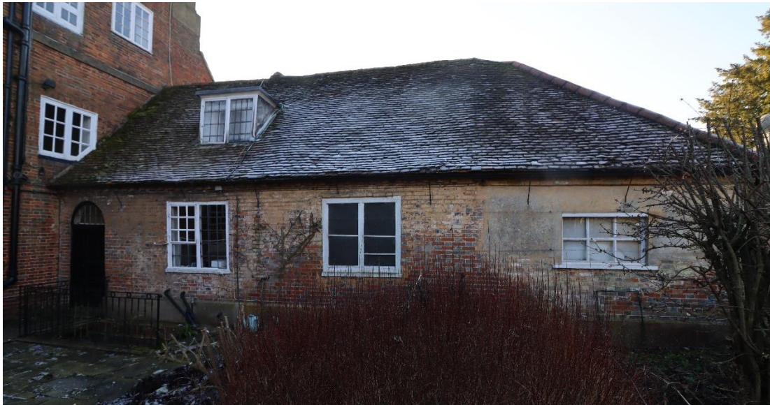
West elevation of service wing
