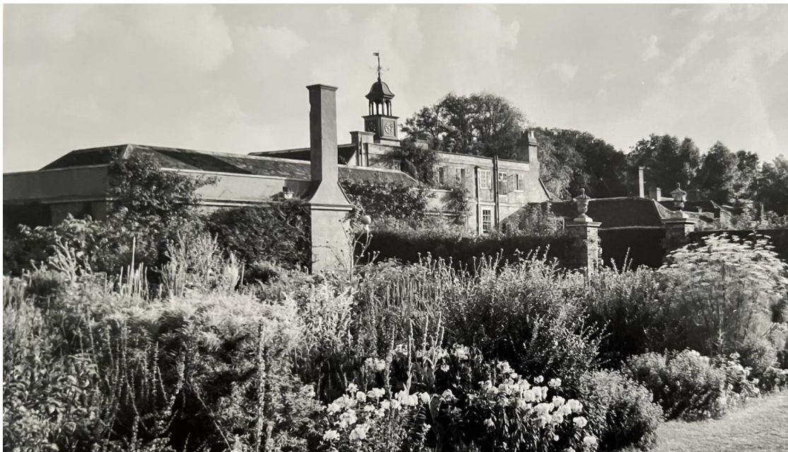
Original Music Room chimney stack
