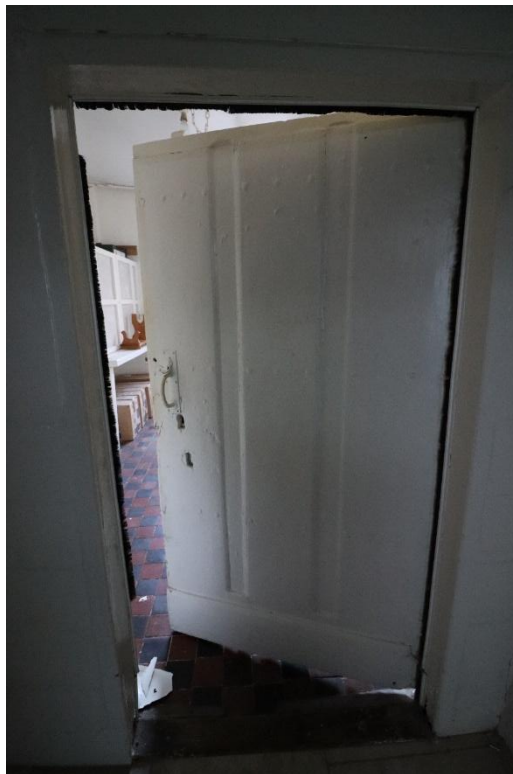
C17th style door to Cold Store to be relocated to new Laundry (Historic recording P 26-27)
