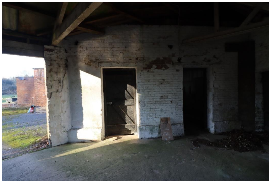
2no external ledge and brace doors (to be retained) to south wall of former Coach House. Door into Store (lhs) to be re-hung.
