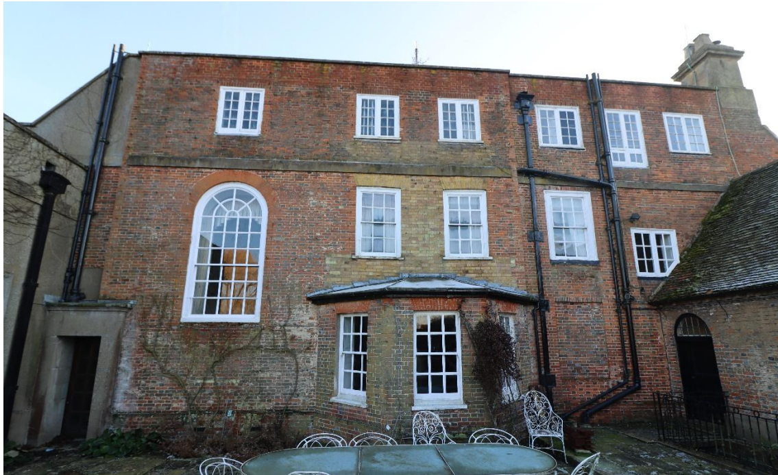
Existing drainage on rear (north) elevation of Villa (to right and left)
