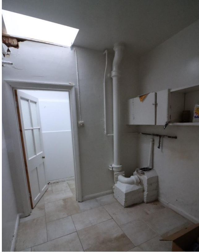
Lobby to Cloakroom. C18th walls to right & left to remain. MC20th door, partition and rooflight to be removed
