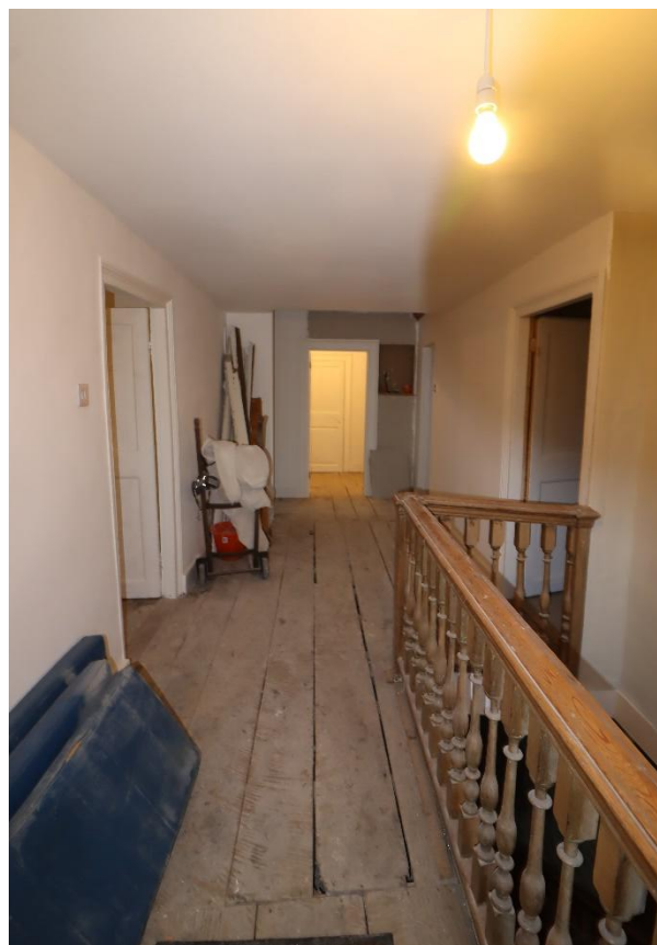
Second Floor Landing
