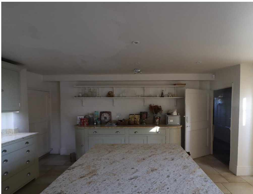
MC20th wall (forming Butler's Pantry) and shelving to be removed
