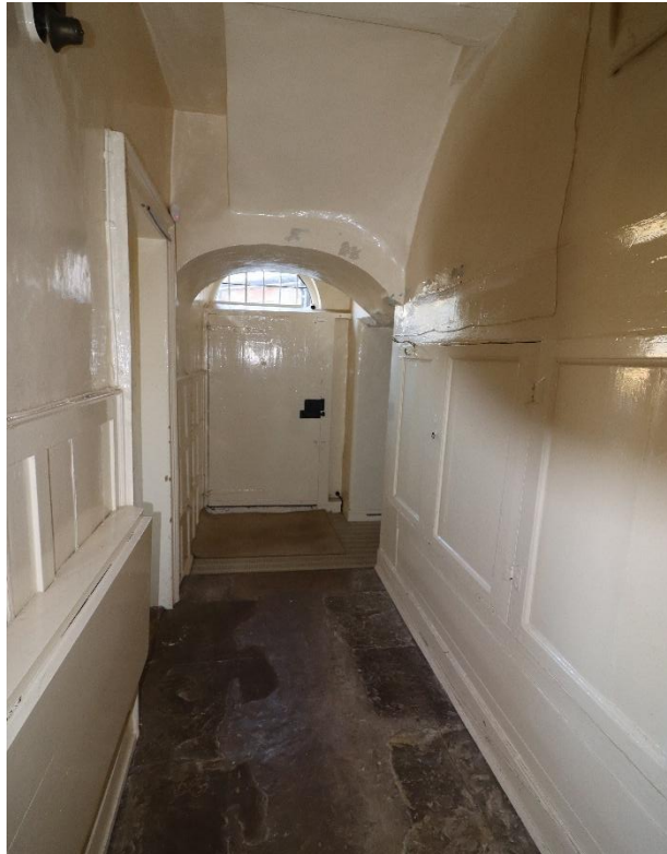
Service Corridor at rear of Main Villa. C17th fireplace behind cupboard doors (rhs)
