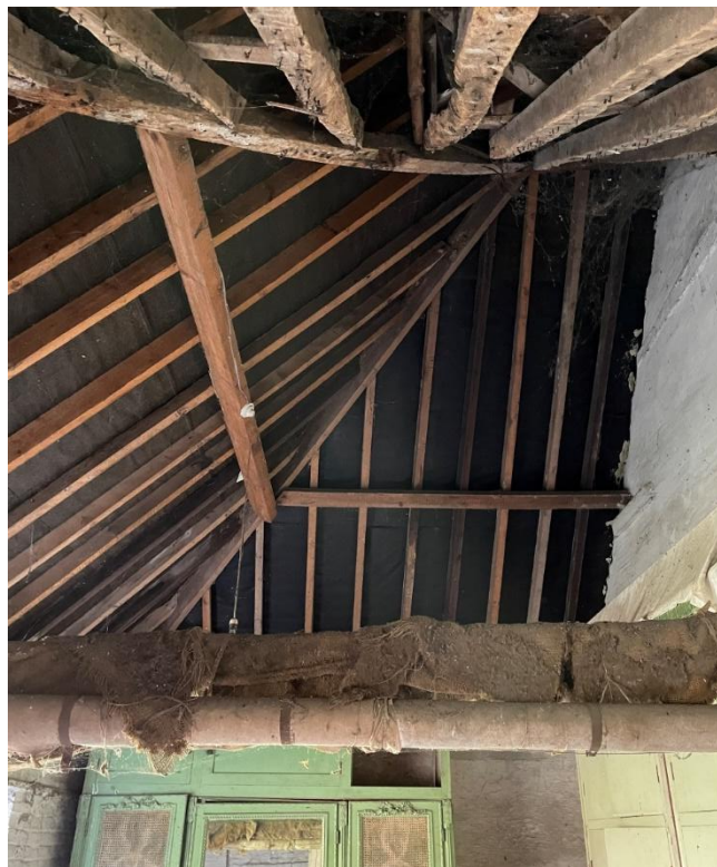
Location above existing store for new floor
