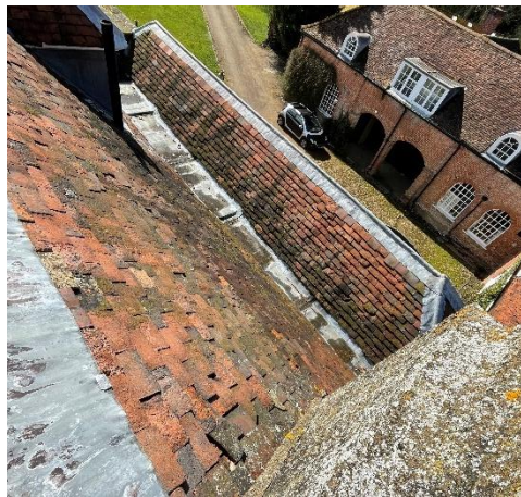
West side stepped valley gutter
