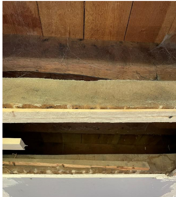
Photo taken in central north room indicating roof build-up. The lower timbers are assumed to be 1939 from works.
