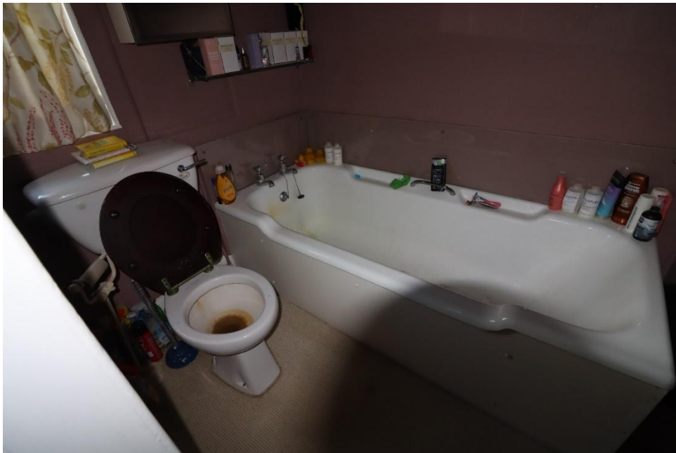
Existing ensuite to Bedroom 2. MC20th sanitaryware, plumbing and drainage to be removed. Room to be converted to a Dressing Room
