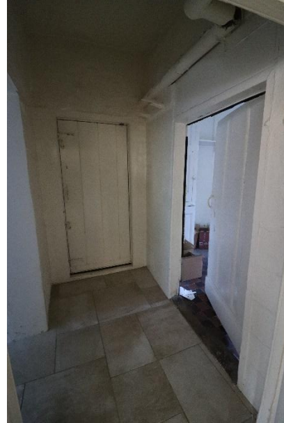
C20 th door to store to be removed
