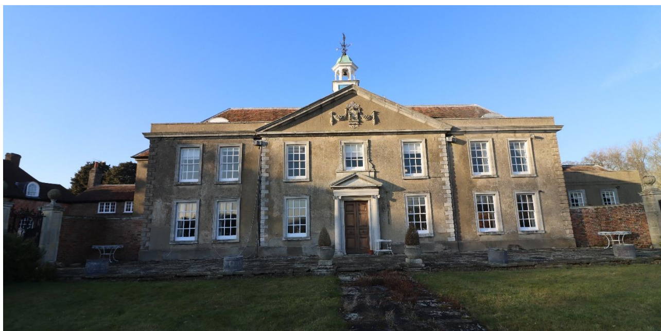
Front Elevation (south) of Main Villa
