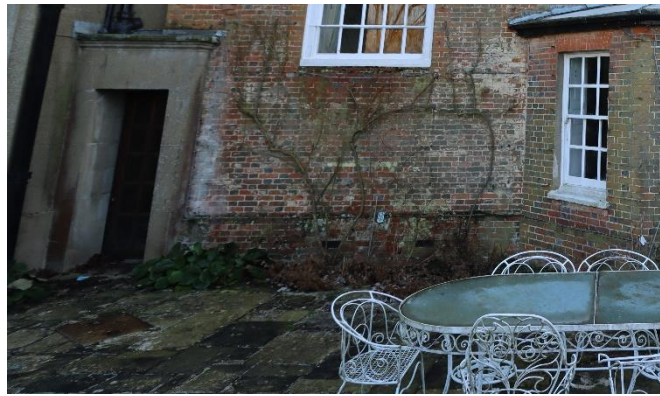
Location of infilled window at low-level
