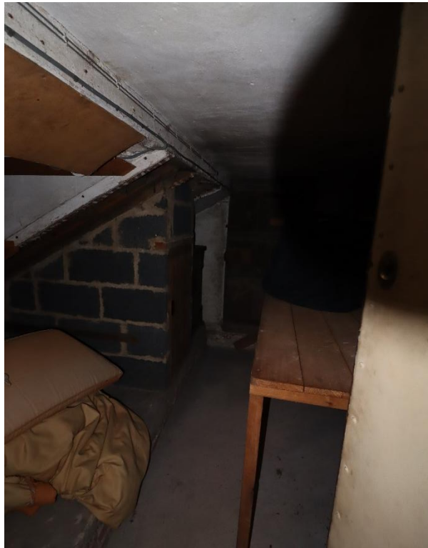
North-west service corridor to be converted to a Cloakroom
