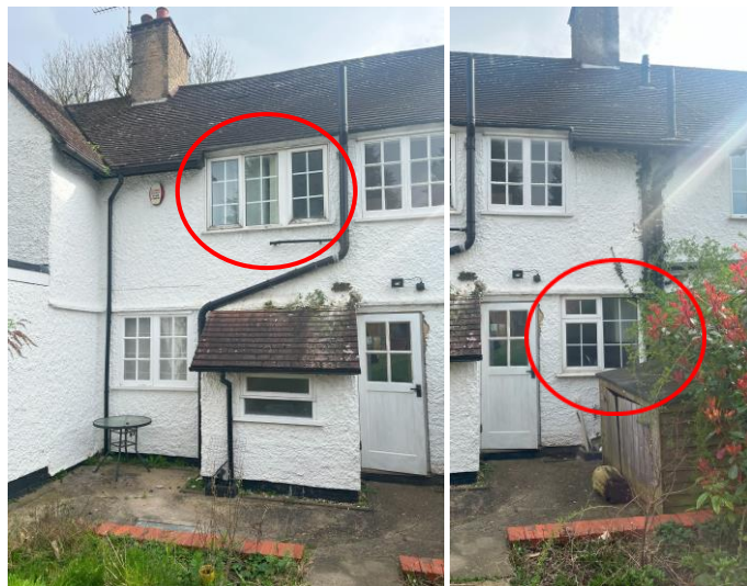
Photos of rear of 21 Lytton Avenue, highlighting uPVC windows to be replaced.
