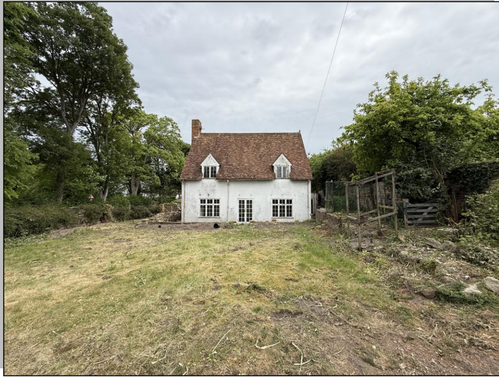
Photograph indicating the rear (west) elevation of the property
