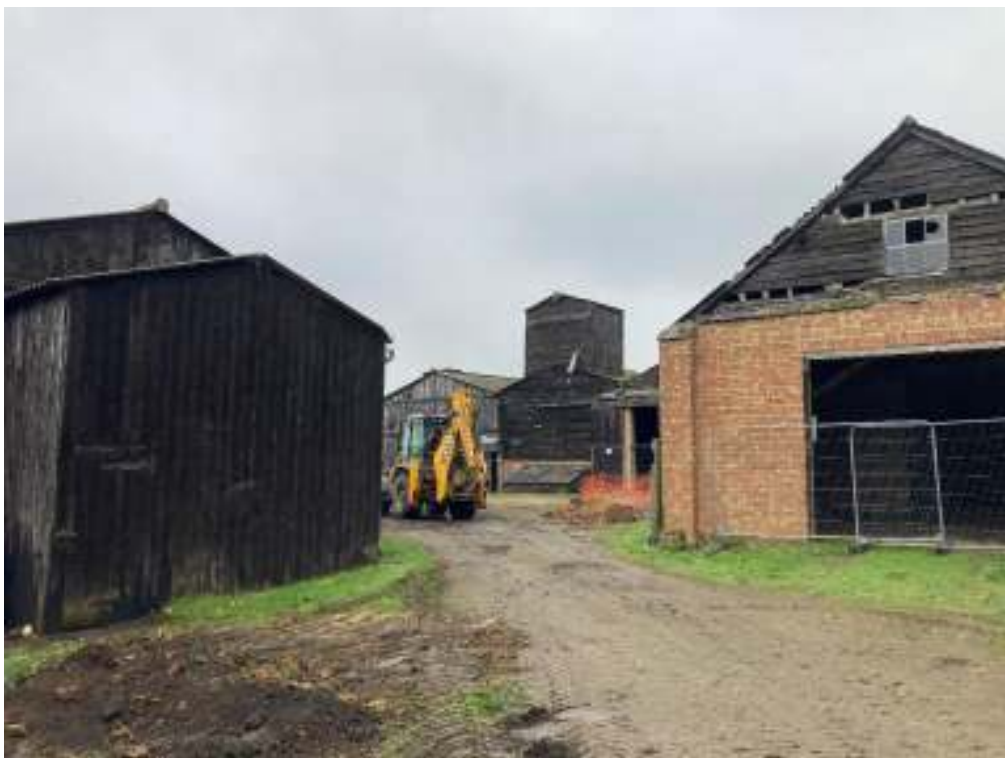
Entrance to courtyard, cart shed on left, grade listed building on the right
