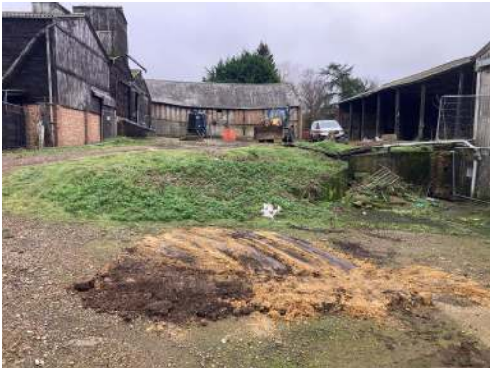
Made-up levels, retaining wall at the right
