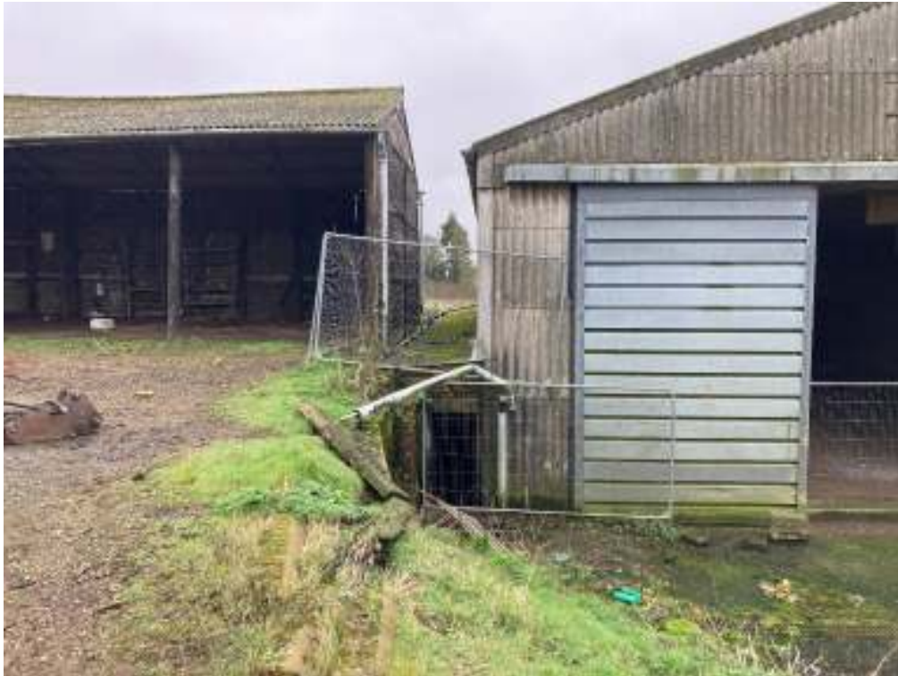
Cart shed on left, adjacent barn on the right (retaining wall at the centre)
