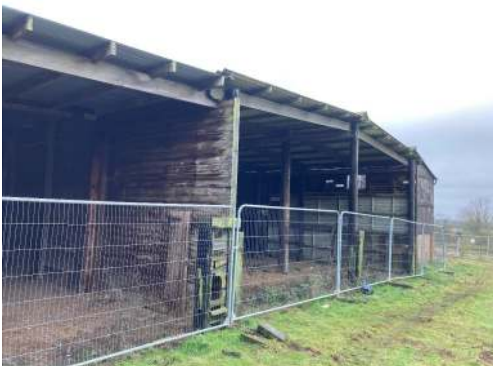
Existing barns adjacent to SA4
