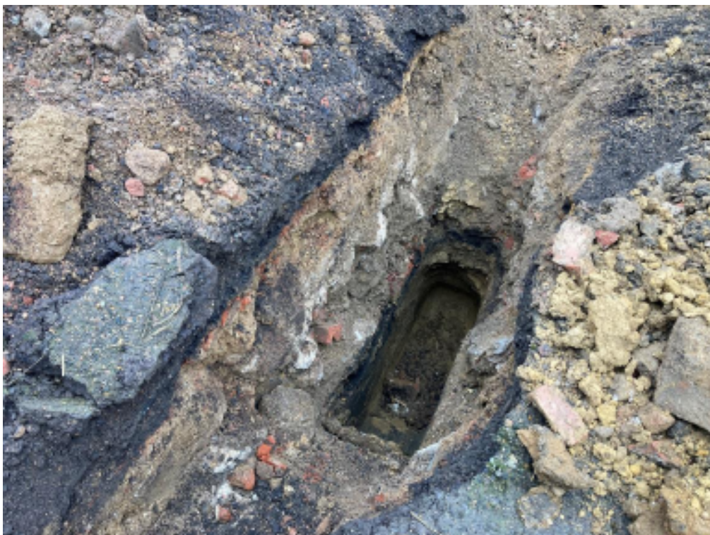
TP1 (deepened Made Ground)
