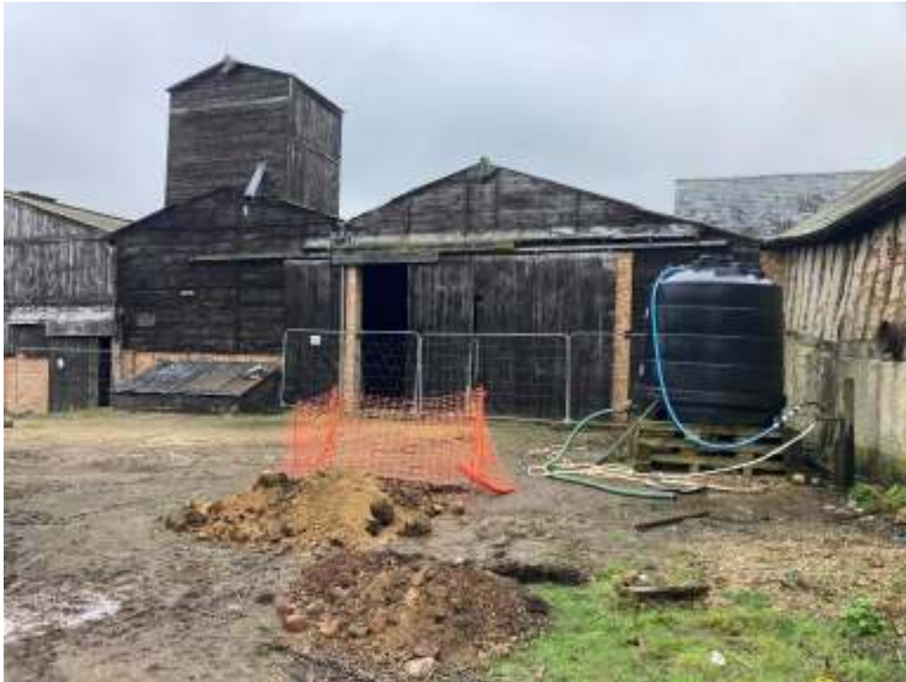
Above groundwater tank and SA1 – granular soils
