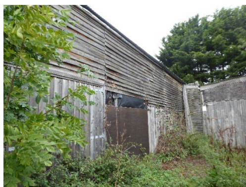
Plate 10: Lifting eastern elevation weatherboarding
