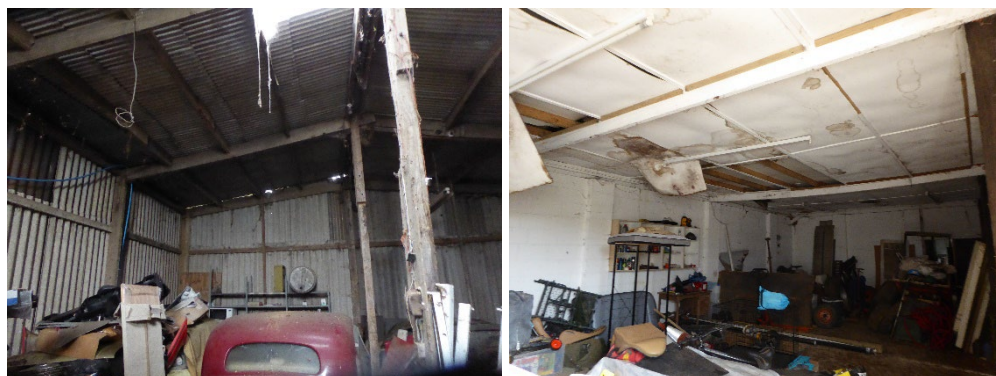
Plates 8 & 9: Internal views of the barn showing lined and unlined walls and roofs
