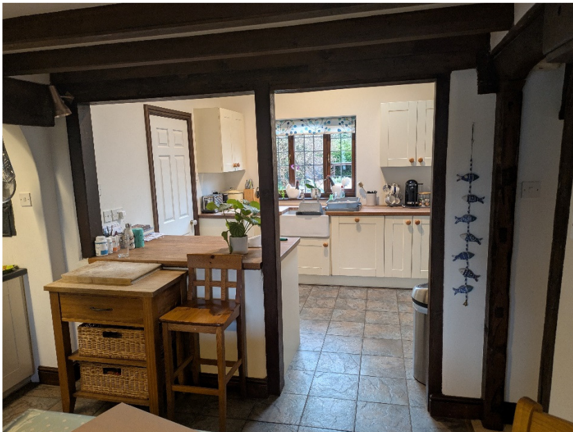
Wall to be infilled with timber studs and plasterboard.
