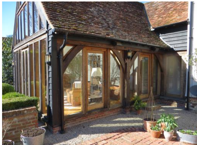
Figure 4.73: Showing the eastern return elevation of the garden room.
