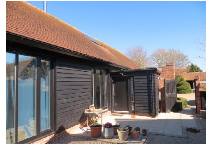
Figure 4.78: Showing the flat roofed porch.
