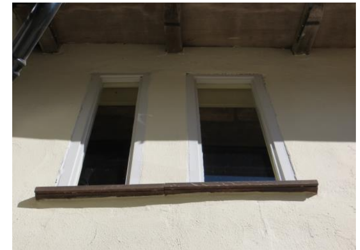
Figure 4.60: Showing the first floor windows at the northern end of the kitchen cross wing.
