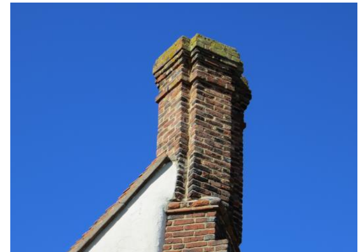
Figure 4.57: Showing the uppermost part of the stack at the southern end of the kitchen cross wing.
