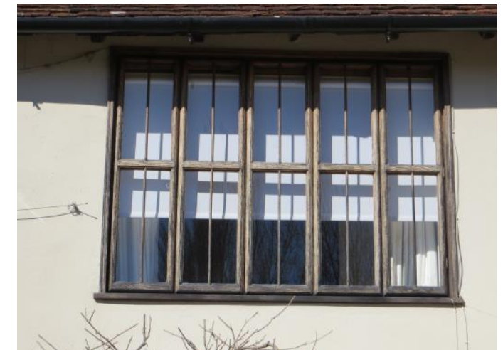
Figure 4.70: Showing the first floor window on the main range.
