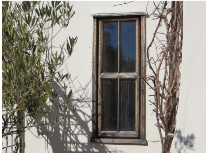
Figure 4.67: Showing the ground window serving the cellar stairs.
