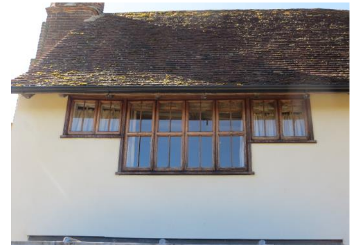
Figure 4.54: Showing the first floor southern window.
