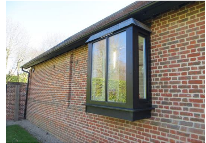
Figure 4.83: Showing the raised bay window on the northern elevation.
