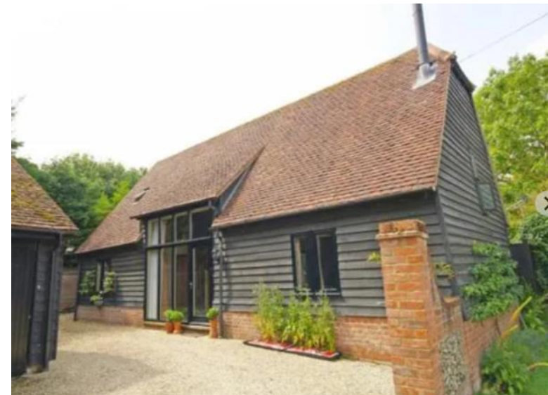
Figure 5.3: Showing the aisled barn north of the Old Manor Farm House (Source: Move Market, n.d.).
