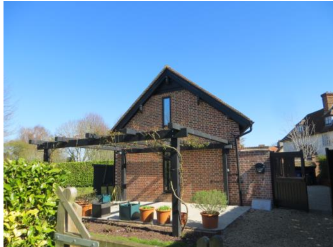
Figure 4.85: Showing the western elevation.
