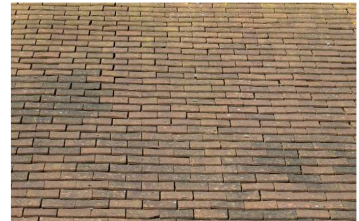
Figure 4.84: Showing the red clay tiled roof covering.
