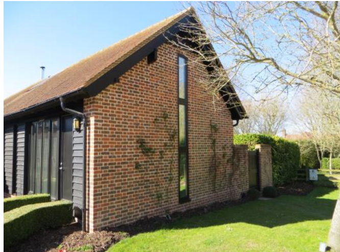
Figure 4.80: Showing the eastern elevation looking north-west.
