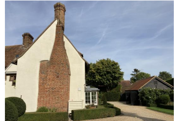
Figure 4.56: Showing the southern elevation of the kitchen cross wing.
