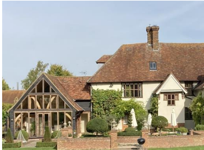
Figure 4.61: Showing the southern elevation of the main range and the garden room.
