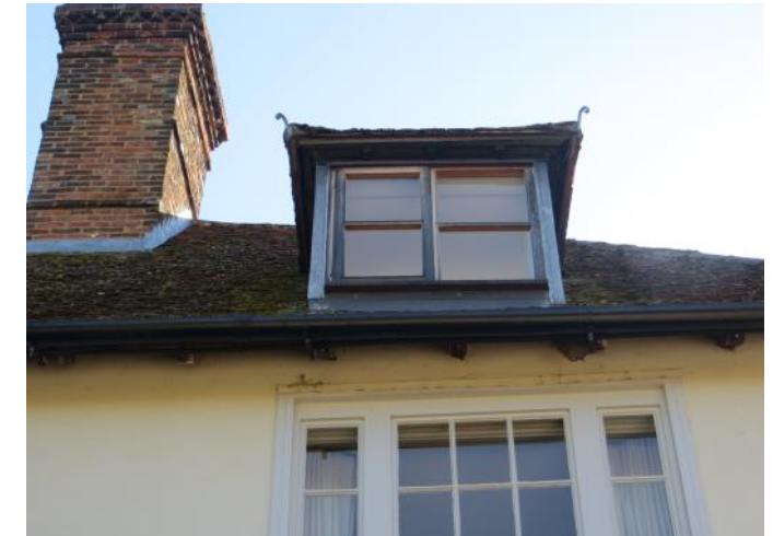
Figure 4.47: Showing the western front dormer.
