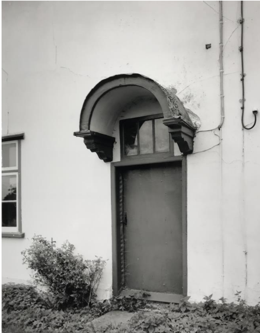
Figure 4.5: 1992-94 photograph (Source: Historic England Archives). Showing the canopy, moulded brackets and door on the main house's northern (front) elevation. Also showing the historic 3-plank door in the main entrance.
