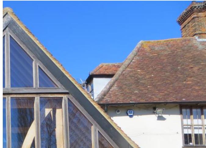
Figure 4.75: Showing the dormer on the main range's western roofslope.
