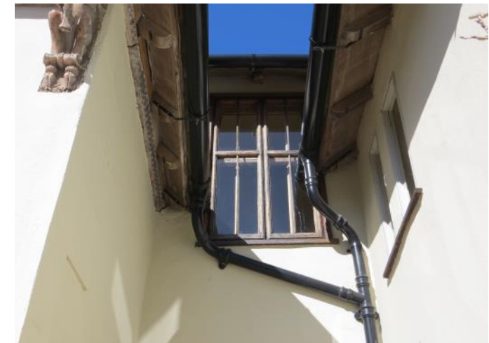
Figure 4.63: Showing the first floor window at the eastern end of the main range.
