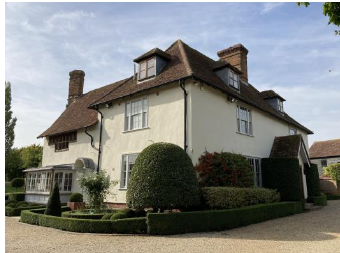
Figure 4.48: Showing the northern and eastern elevations.
