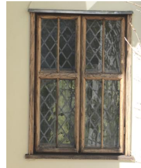
Figure 4.62: Showing the eastern ground floor window on the main range.
