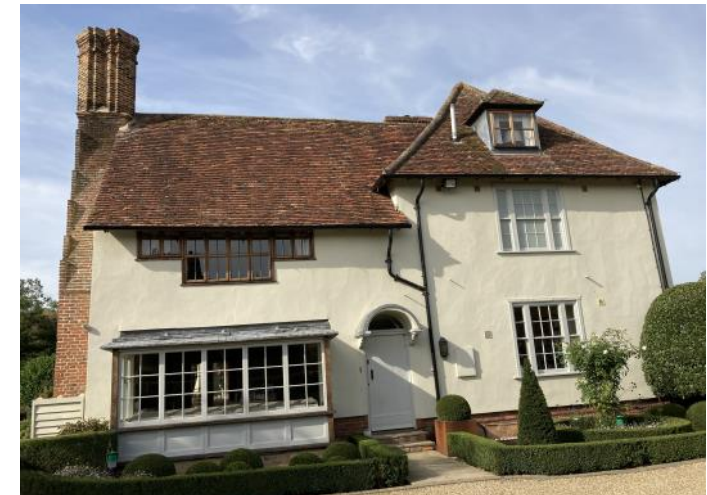
Figure 4.49: Showing the eastern elevation.
