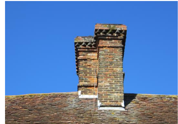
Figure 4.72: Showing the corniced stack in the centre of the main range's roof.
