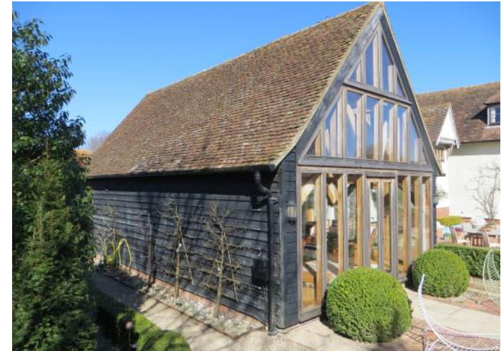
Figure 4.76: Showing the western and southern elevations of the garden room.
