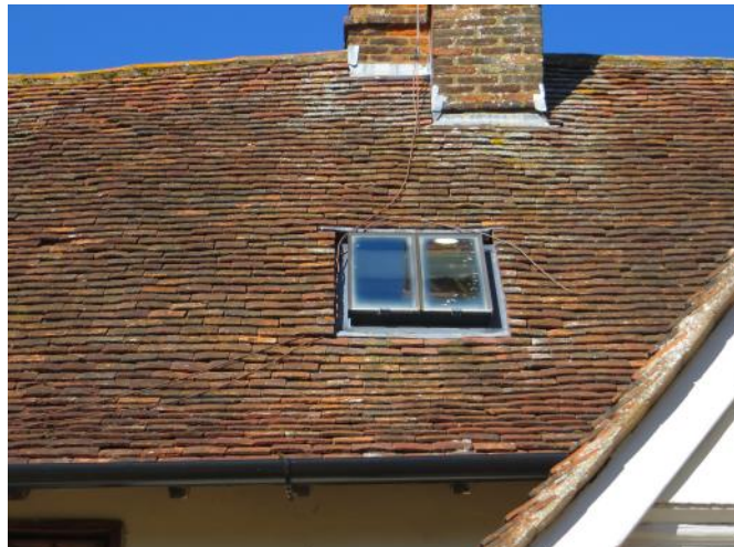
Figure 4.71: Showing the conservation rooflight on the main range's southern roofslope.
