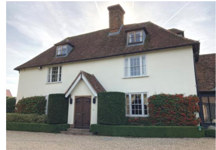
Figure 4.42: Showing the northern (front) elevation.
