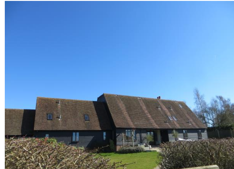
Figure 5.2: Showing the aisled barn and sheds south west of the Old Manor Farm House.
