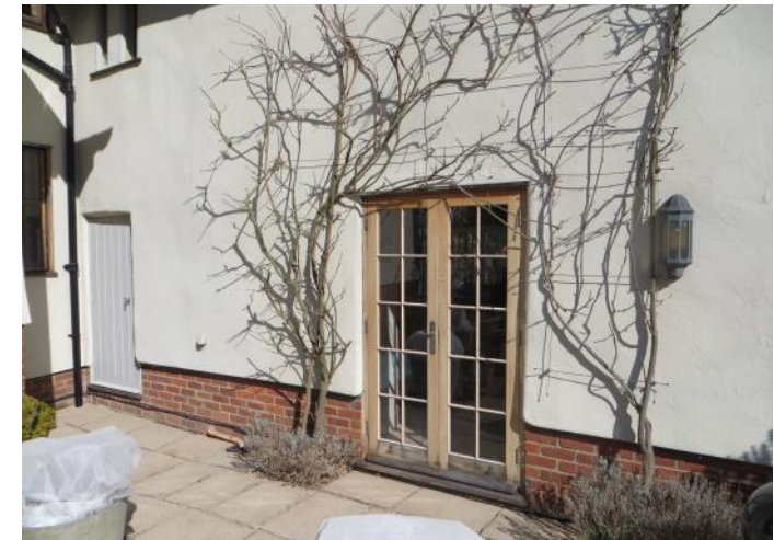
Figure 4.59: Showing the French windows installed on the western elevation of the kitchen cross wing.
