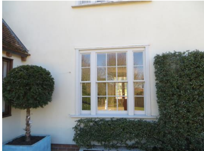
Figure 4.44: Showing the western ground floor window.
