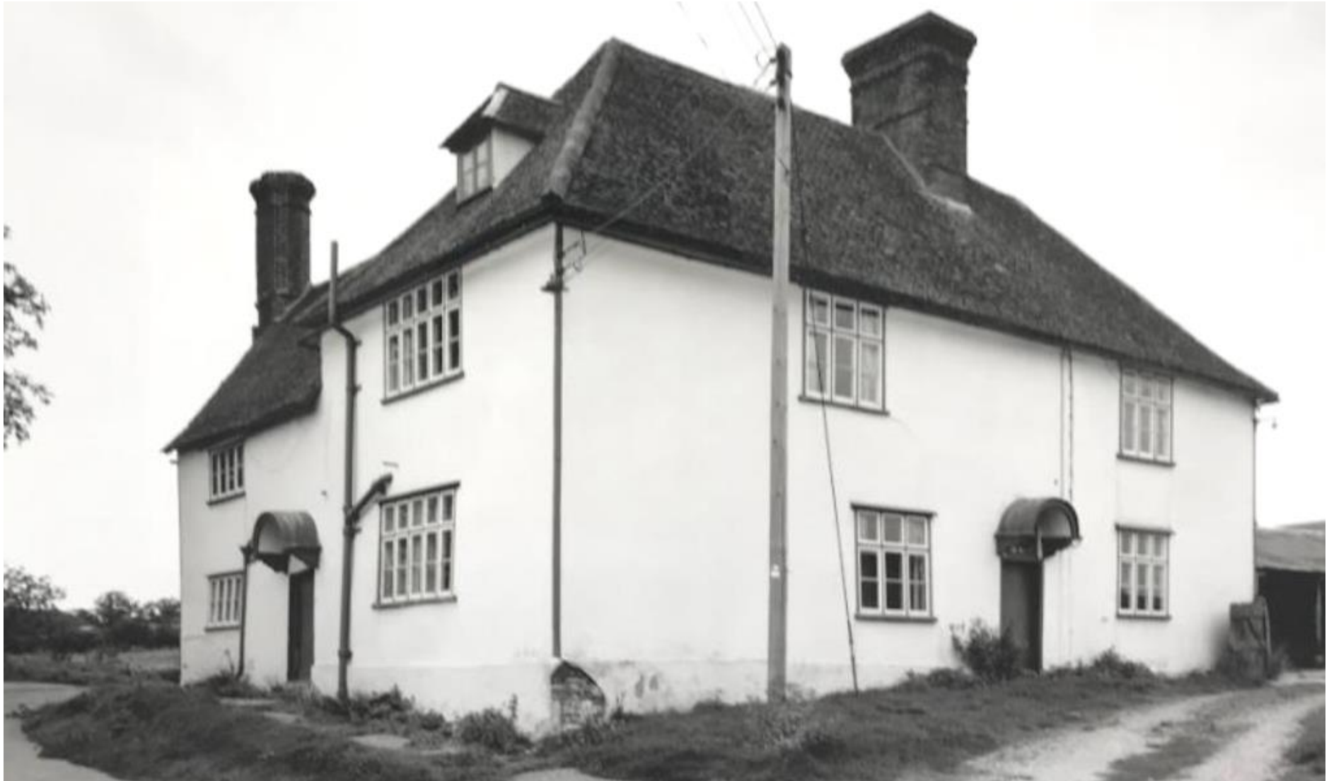
Figure 4.4: 1992-94 photograph (Source: Historic England Archives). Showing the main house's northern and eastern elevations.
