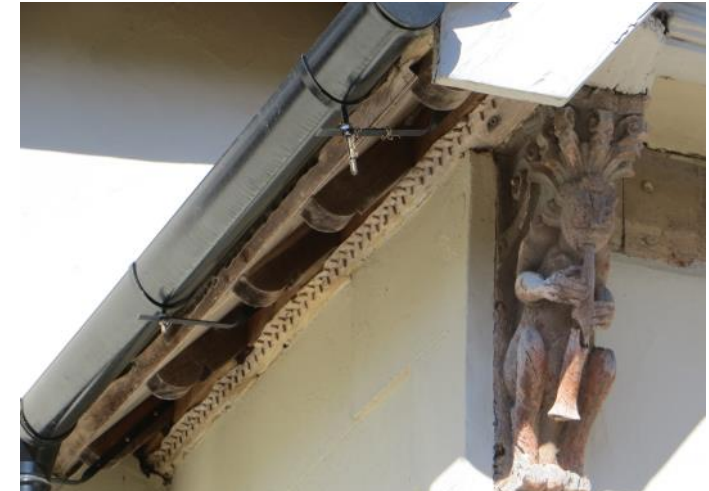
Figure 4.65: Showing dentilled cornice on the western elevation of the stair wing. Note the carved satyr.
