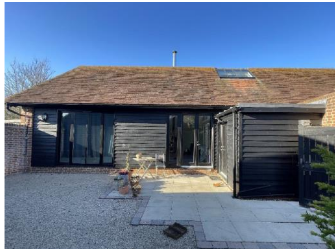
Figure 4.77: Showing the western part of the southern elevation.
