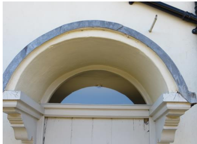
Figure 4.50: Showing the renewed canopy on the eastern elevation.
