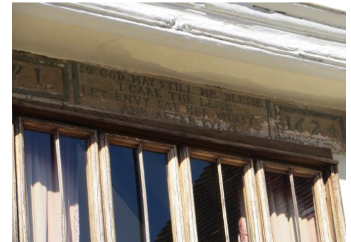
Figure 4.66: Showing the inscription above the first floor window on the stair wing.
