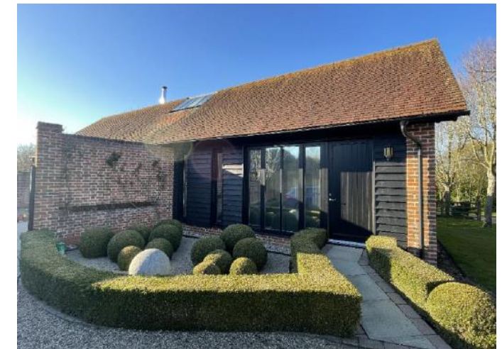
Figure 4.79: Showing the eastern part of the southern elevation.
