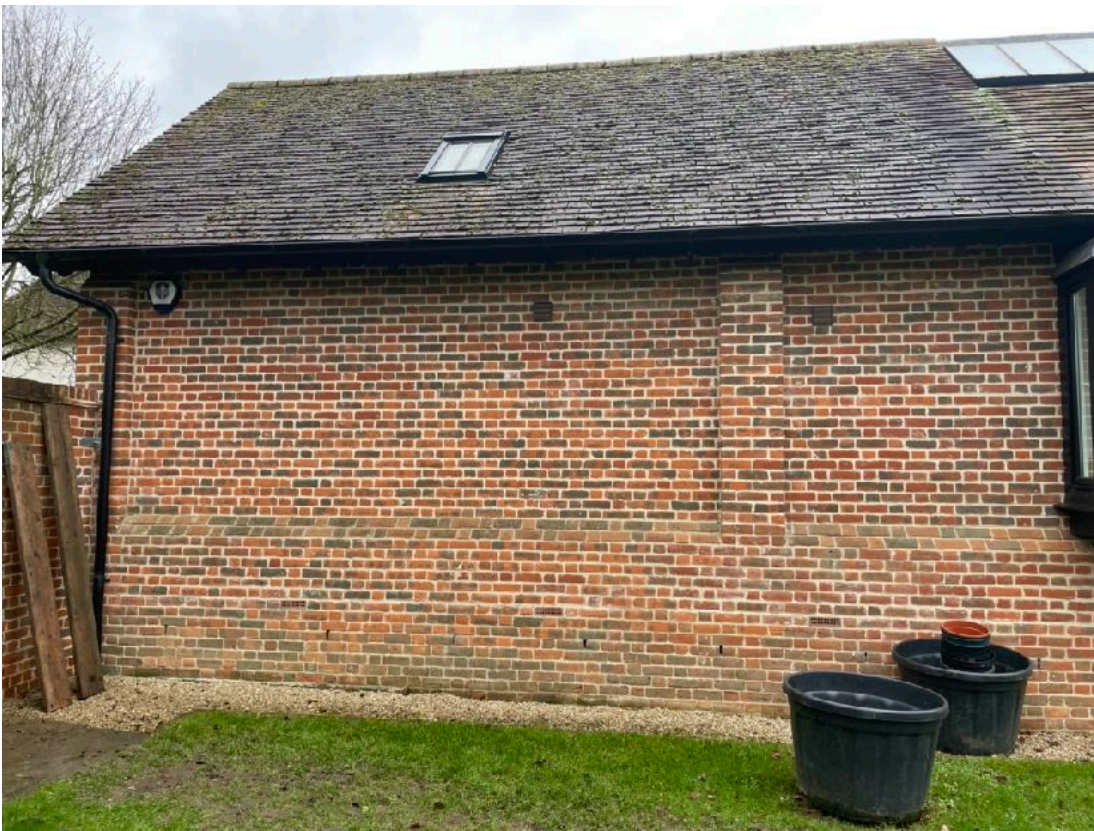
Detail of existing brickwork wall
