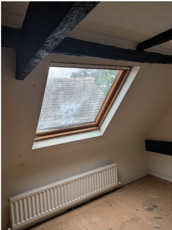
Velux windows to be replaced.
