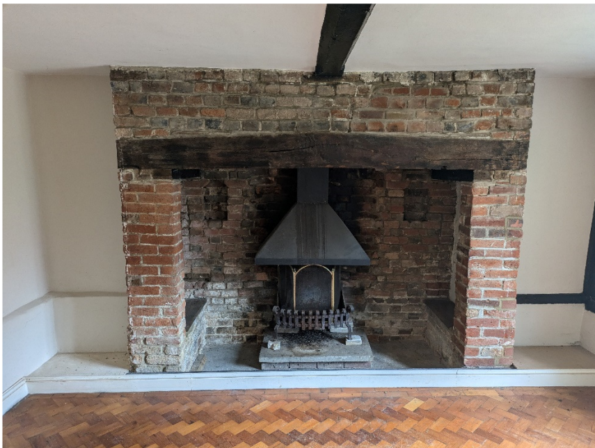
Fire to be replaced all brickwork to remain no alterations to the structure
