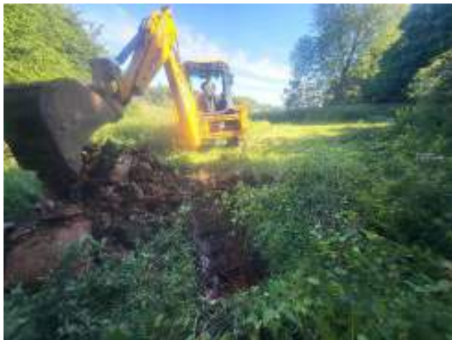
Photo 1: TP1 being excavated with JCB
