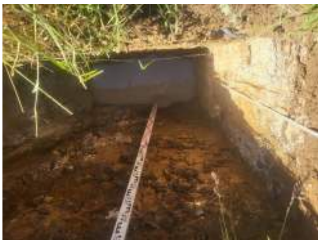
Photo 3: TP2 filled with water
